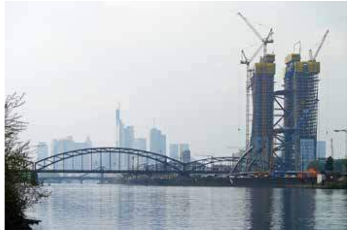
European Central Bank new building under construction Frankfurt Germany.
